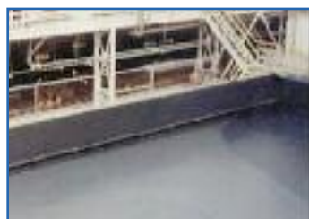
Bund after relining
